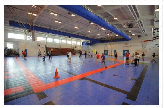
**Situation** > Lake County Schools Gymnasium A/C renovation project for Oak Park Middle, Clermont Middle and Clermont Elementary schools. The scope of work consisted of demolition, fabrication/installation of duct work, new conduits, installation of new motorized dampers, new fire alarm, new electric, installation of chain link fence and gates.
